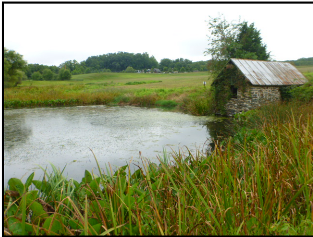
1. Old stone springhouse. View is south.
