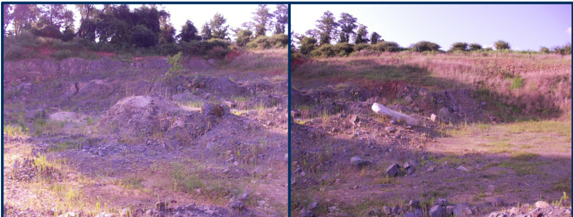
Photo 7.5 - Representative Photos of Borrow / Waste Pit, adjacent to Site B.
