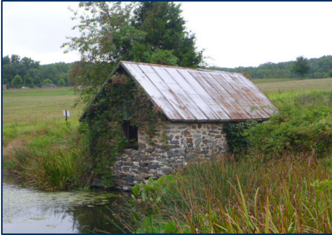
Photo 8.11 - Springhouse at the Edgeley Grove Farm Pond at Site A
