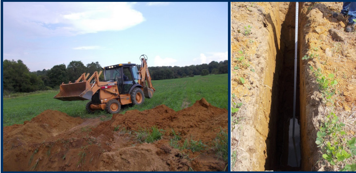
Photo 7.2 - Site A Test Pit Excavator and Sample Test Pit
