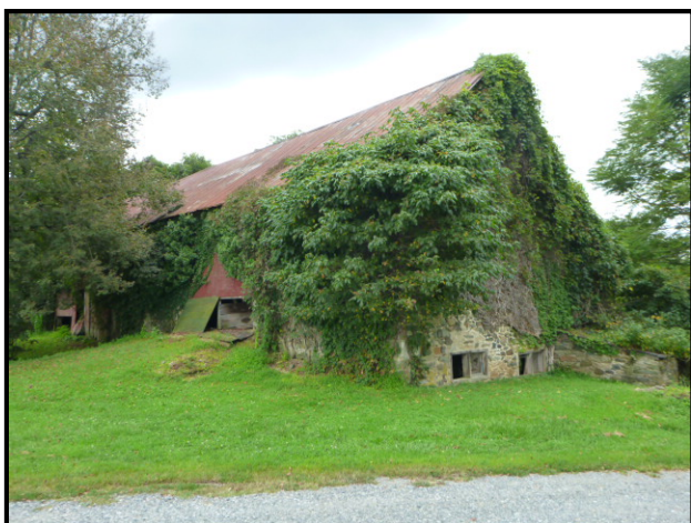
11. Old barn. View is south; barn will not be impacted.
