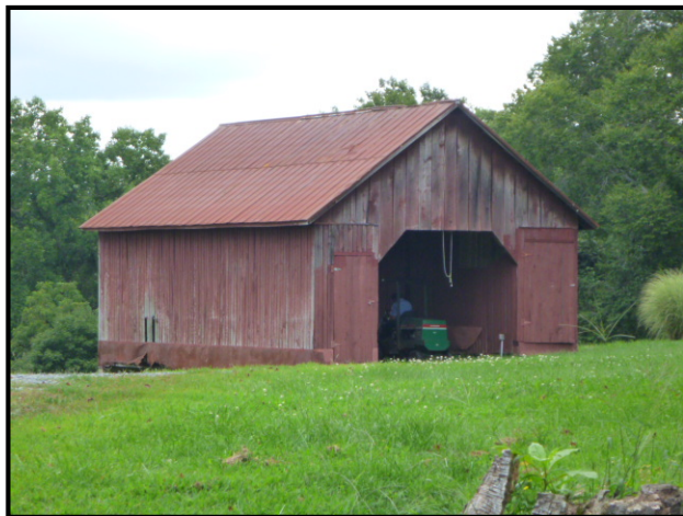
12. Old barn. View is east; barn will not be impacted.
