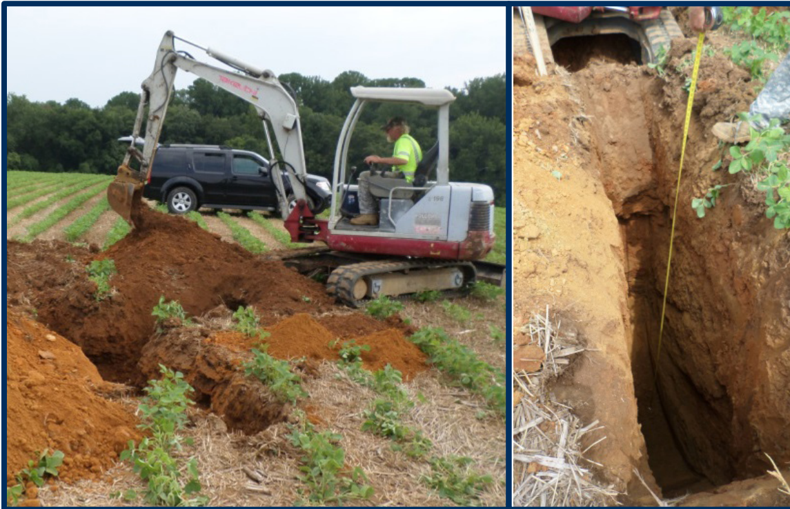
Photo 7.3 - Site B Test Pit Excavator and Sample Test Pit
