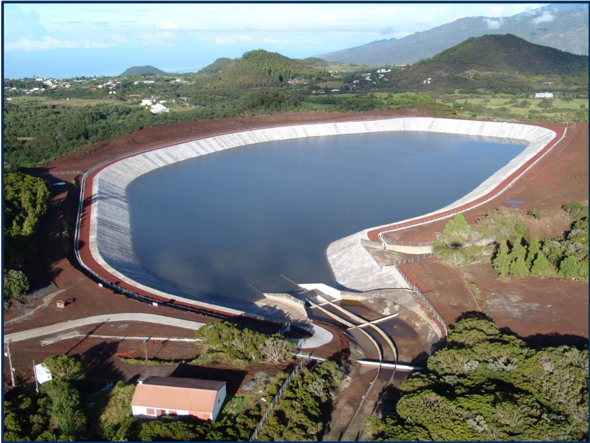
Photo 4.1 - Example of Lined Reservoir, Courtesy of Carpi USA Inc.
