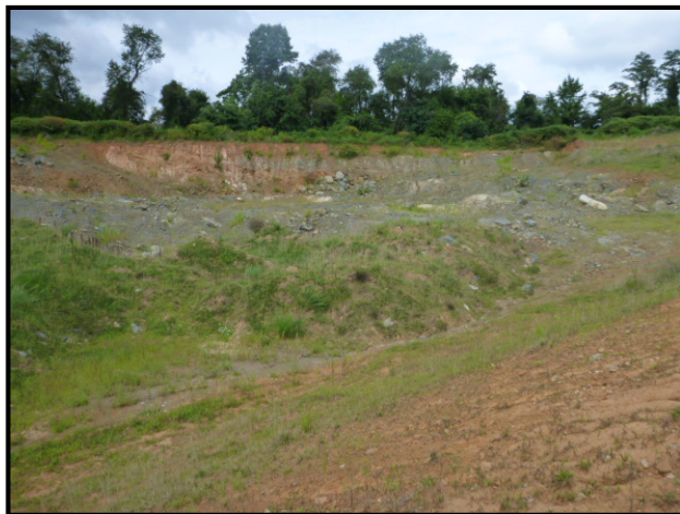
10. Rock and top soil borrow pit. View is west.
